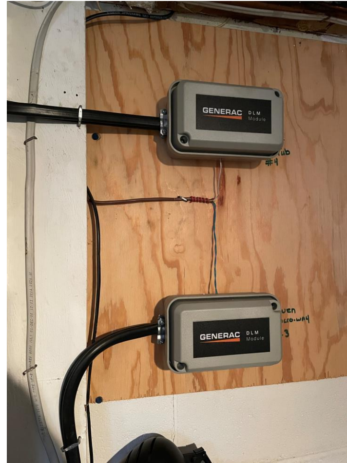
2 OF 4 LOAD SHEDDING RELAYS
