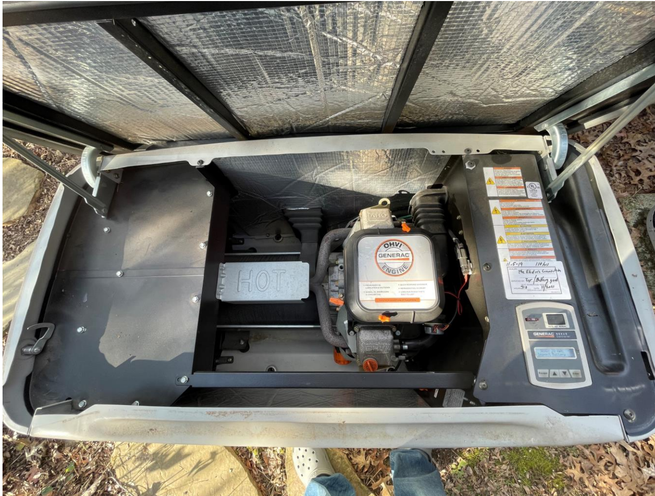
ENGINE-GENERATOR COMPARTMENT
