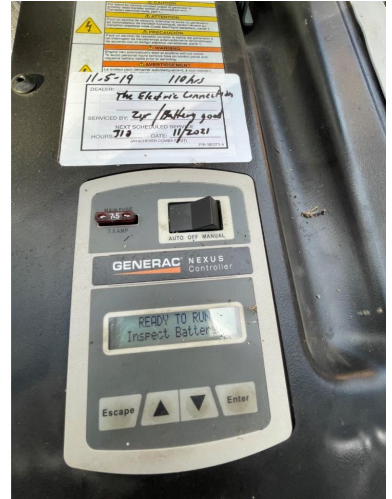
MICRO-CONTROLLER AND PANEL CONTROLS
