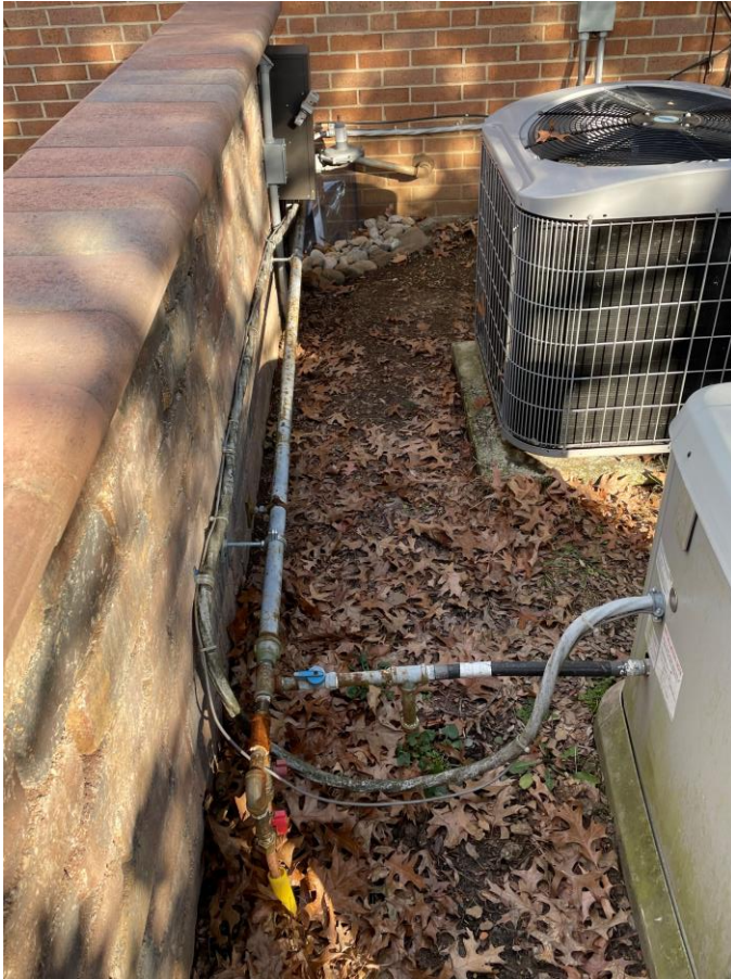
GAS LINE & GENERATOR AC OUTPUT
